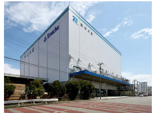
Kawasaki Refrigerated Warehouse
